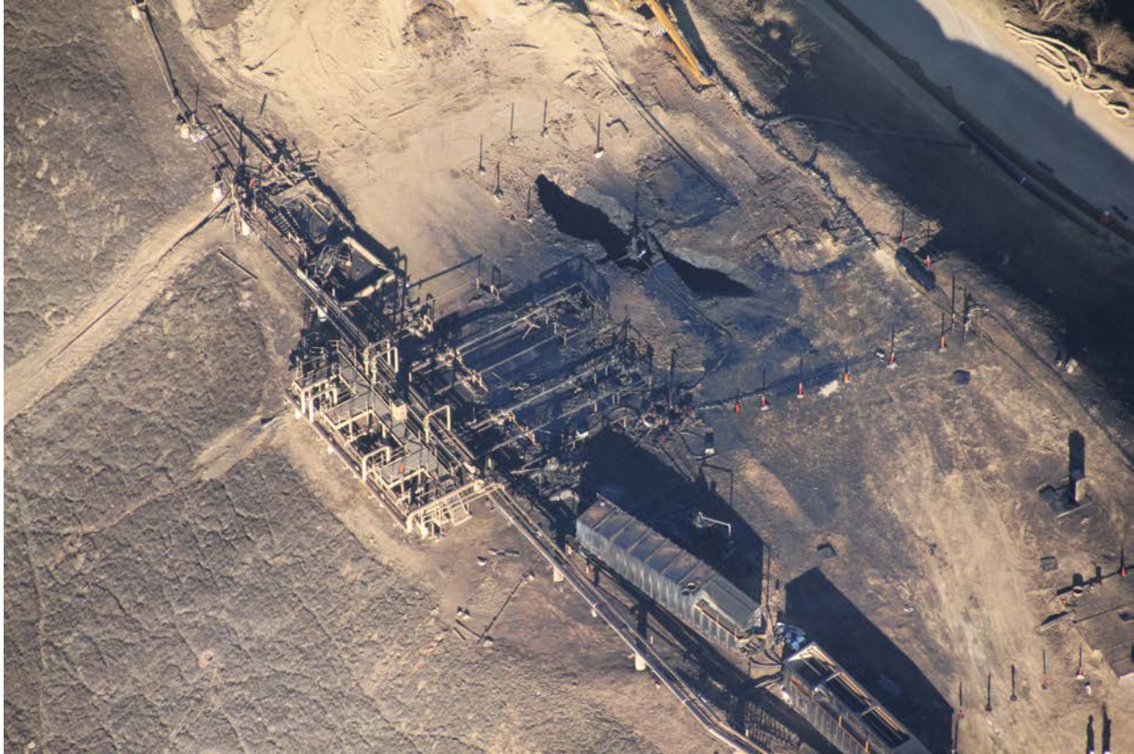
Figure 3. The Aliso Canyon gas storage facility methane leak cost the well operator approximately $763 million in response costs, displaced over 5,790 families, and released the equivalent GHG emissions of a half-million cars.
